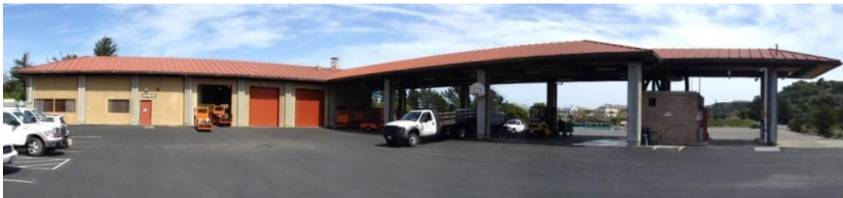
Maintenance Building with standing seam metal roofs
