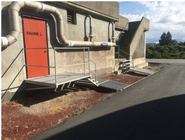
Stair modifications to account for settlement
