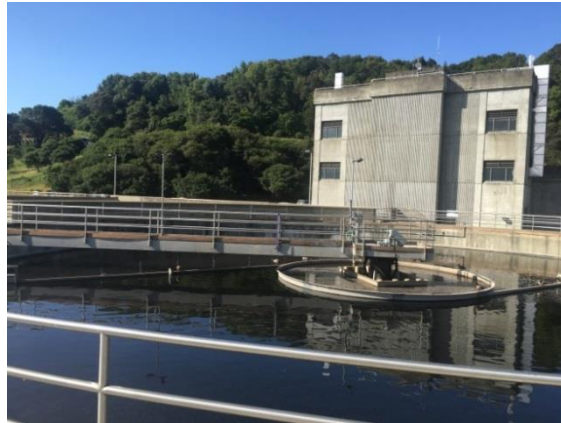
Secondary clarifier in operation
