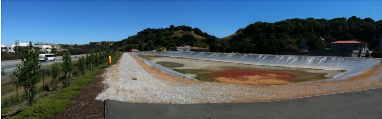
Effluent Storage Pond
