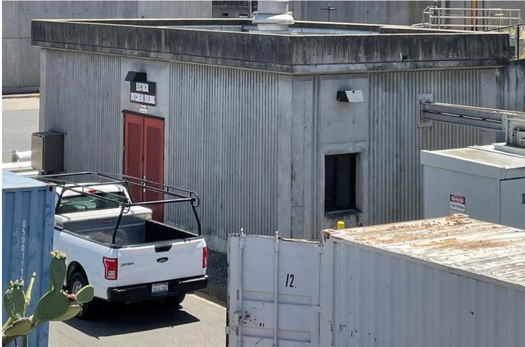
Switchgear building and transformer
