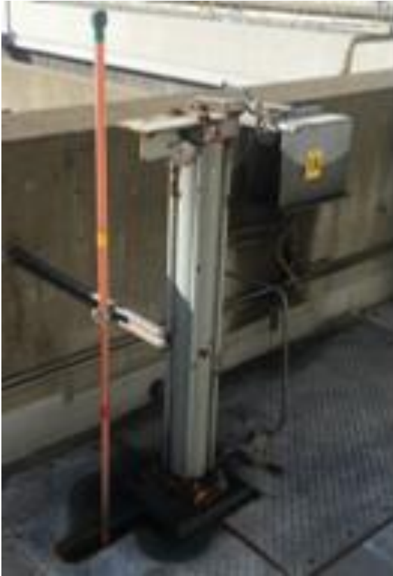
Hydraulic gate actuator
